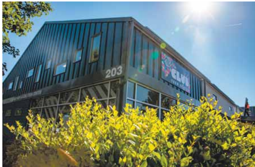
The Boys & Girls Club in Grants Pass received a grant from Pacific Power to pay for the solar panels that were installed on the roof of the facility.
